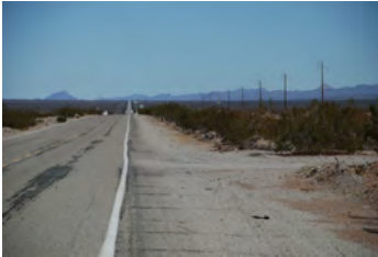
Figure 158 View east from Danby Rest Area
