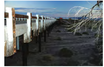
Figure 162 Timber trestle bridge at Avon Wash
