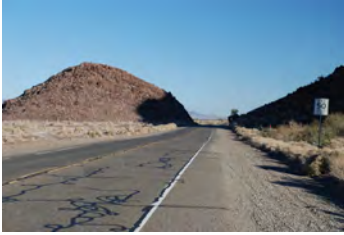
Figure 157 Route 66 approaching Newberry Springs eastbound
