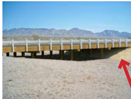
Figure 175 Simulation showing proposed 'W' shaped guardrail painted white (courtesy of San Bernardino County DPW); note post caps will also extend above the 'W' beam
