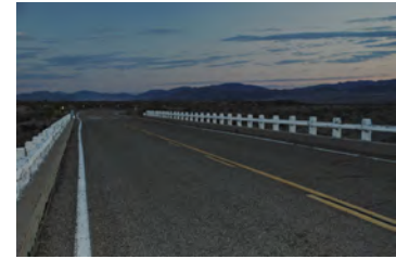
Figure 172 Existing (and original) timber bridge railing
