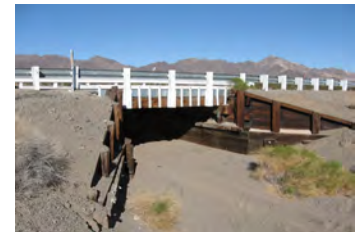
Figure 163 View of bridge rail and abutment walls at Amboy bridge
