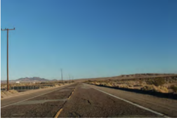
Figure 176 Rough pavement between Newberry Springs and Ludlow limits the potential for bicycle-based heritage tourism.
